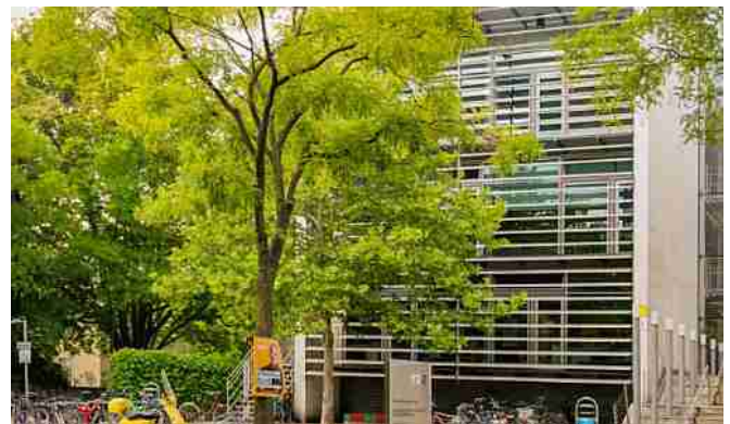
Brise Soleil System, MTZ Dresden
